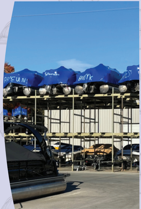
Upland/Dry stack storage of boats
